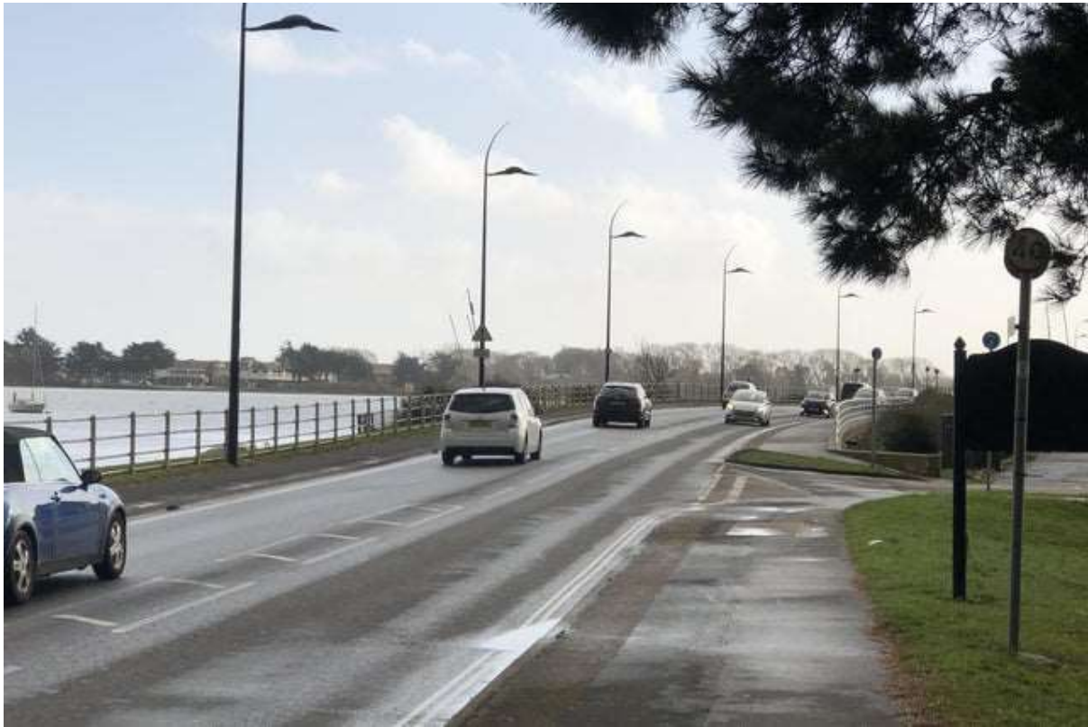
Langstone Bridge, the only road on and off Hayling Island. Picture: Chris Moorhouse Copyright: JPIMedia
